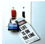
Switch lock and tag
